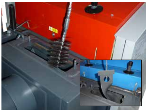
Sample of cleaning of the flue way with a wire brush - upper lid. Remove flue gas brake (turbulators) during cleaning.
