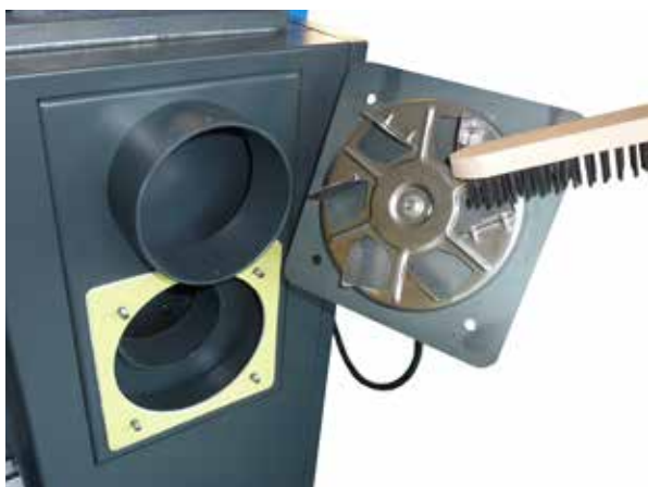
Sample of cleaning of impeller and checking uprightness of vane on exhaust fan
