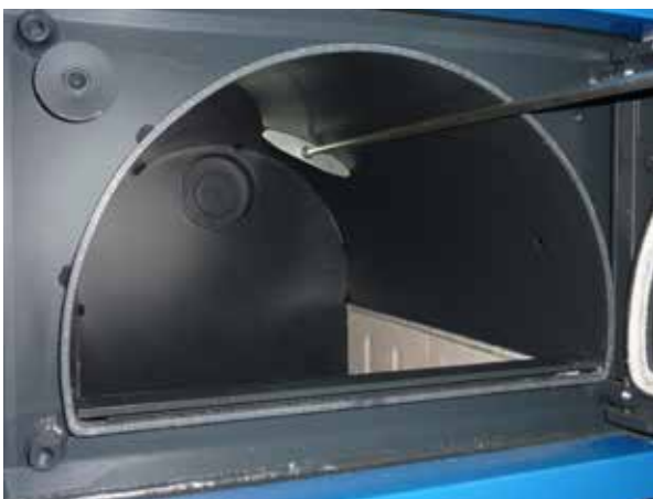
Cleaning the upper stoking chamber with the scraper (poker)
