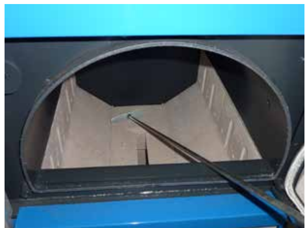
Sweeping the ash through the nozzle down into the bottom (cleaning) chamber. The opening in the nozzle must be always clean and free.
