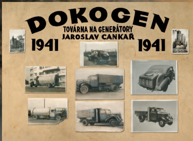
Wood-gas fuel generator DOKOGEN
